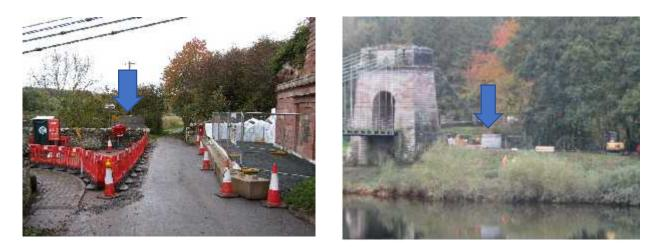
The photographs above show the two concrete drums (arrowed) which will be used as foundations/anchors for the cable apparatus; one on private land on the English side (*left, 23 Oct*), the other on the riverbank footpath on the Scottish side (*right, 21 Oct*)
