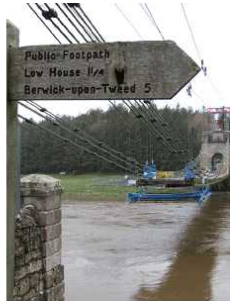
Above: left and right : 27 th January Deck timbers being removed to the English side by Woodliner cable crane.
