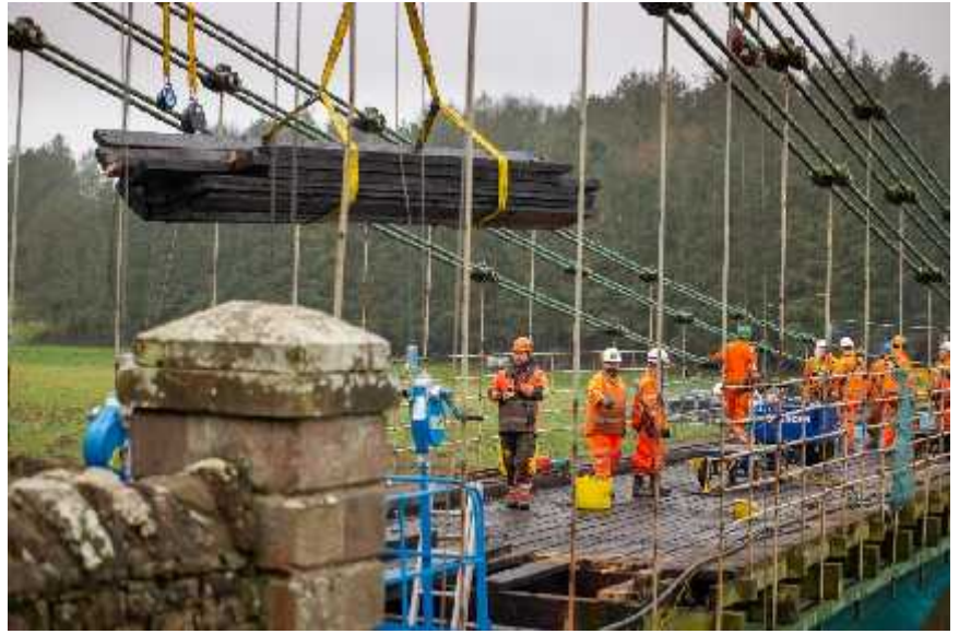
Above: left and right : 27 th January Deck timbers being removed to the English side by Woodliner cable crane.
