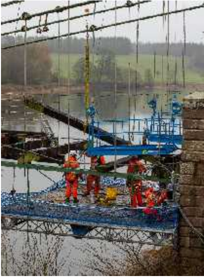
Above: left and right : 27 th January Deck timbers being removed to the English side by Woodliner cable crane.
