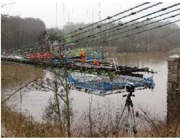
Above: left and right : 27 th January Deck timbers being removed to the English side by Woodliner cable crane.
