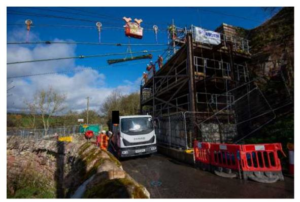
On the 26th March 2021, the Woodliner cable crane lowers a bundle of dismantled chains on to a waiting wagon on the English side of the Bridge, next to the temporary access and accommodation tower, for refurbishment at Spencers' depot.
