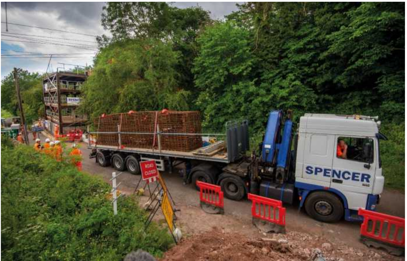
June 17 th 2021 – The English -side rebar reinforcing cage is delivered.
